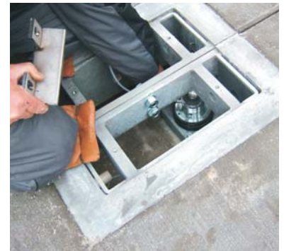
The load cells are mounted.
