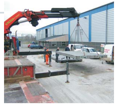
The panels are placed on foundations.
